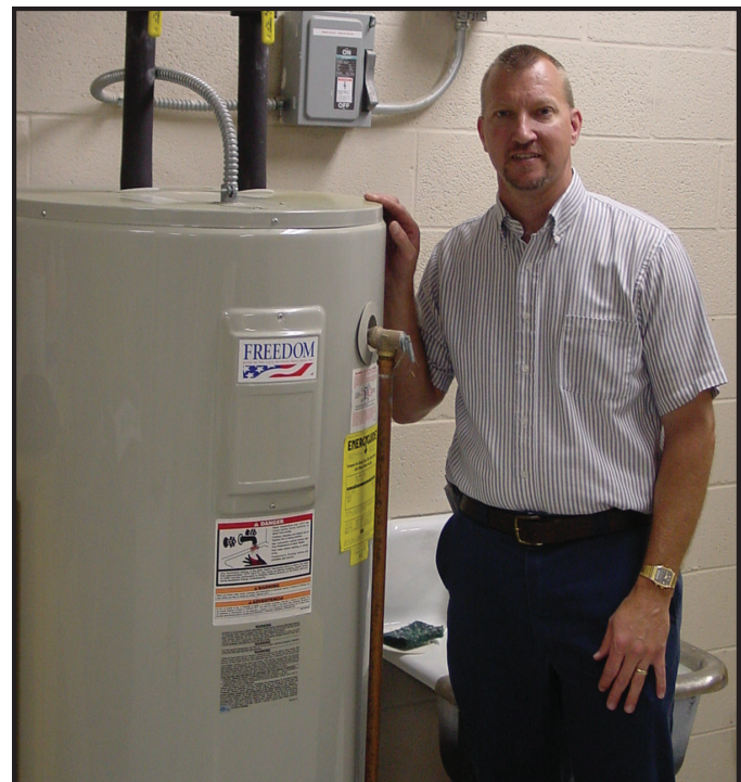
Senior Staff Engineer Brian Shearer looks over the cooperative's load control water heater switch, now known as U-Shift, U-$ave. The program was instituted in 1987 and has saved the cooperative (and co-op members) millions in avoided power purchases.
