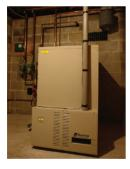
**Heat Pump Plus:** The Heat Pump Plus system combines an air-source electric heat pump and an interruptible electric thermal storage (ETS) unit. Ceramic bricks inside the ETS booster are heated electrically, off-peak. The ETS acts as a backup to the heat pump when the outside temperature drops below a certain point. It also monitors the temperature of the discharging air to assure maximum comfort.
